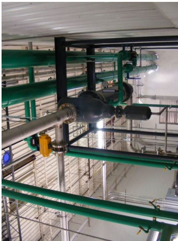
A pipeline-style aftercooler mounted in customer piping (Credit: Alnitak3).
