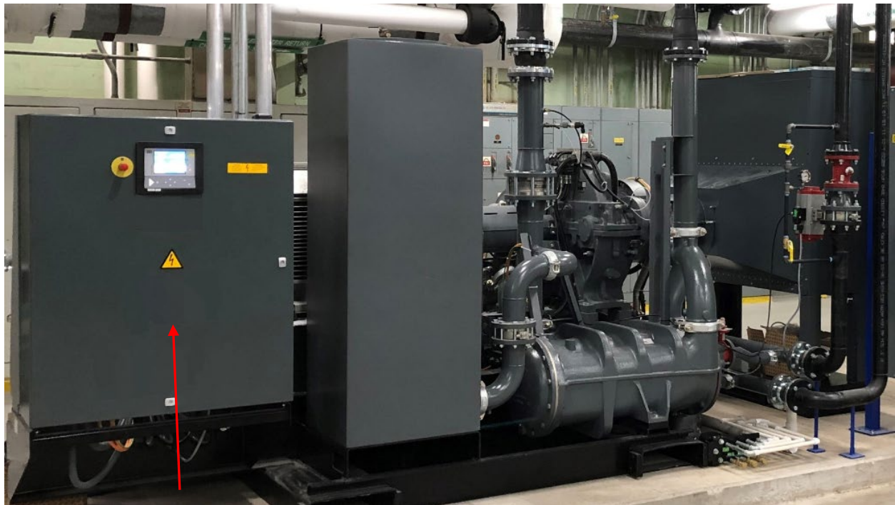
Advanced microprocessor controls minimize surge events
