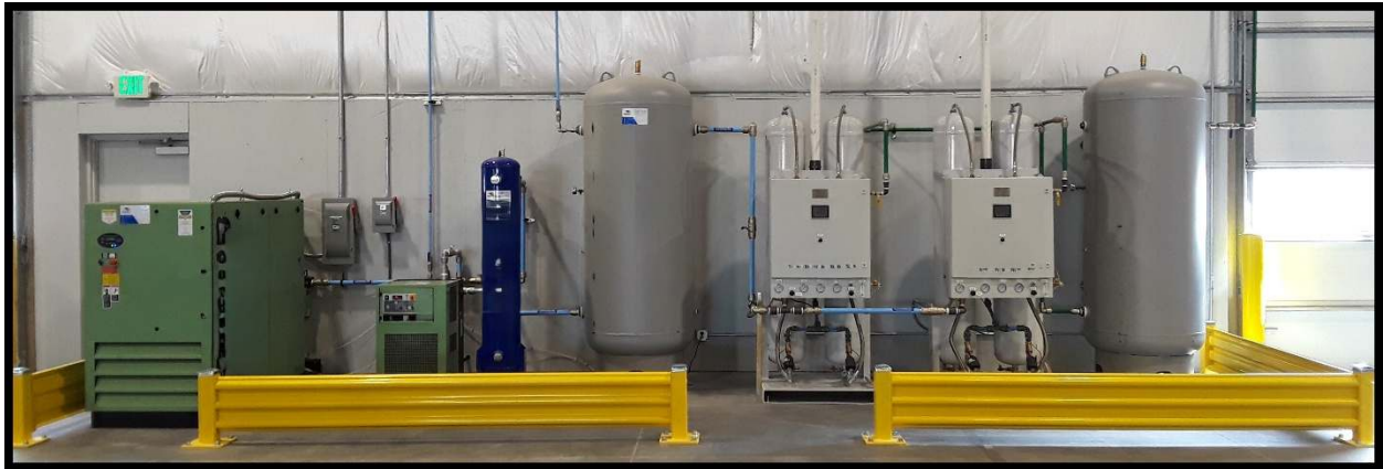
Complete nitrogen generation package with compressor and generator.
