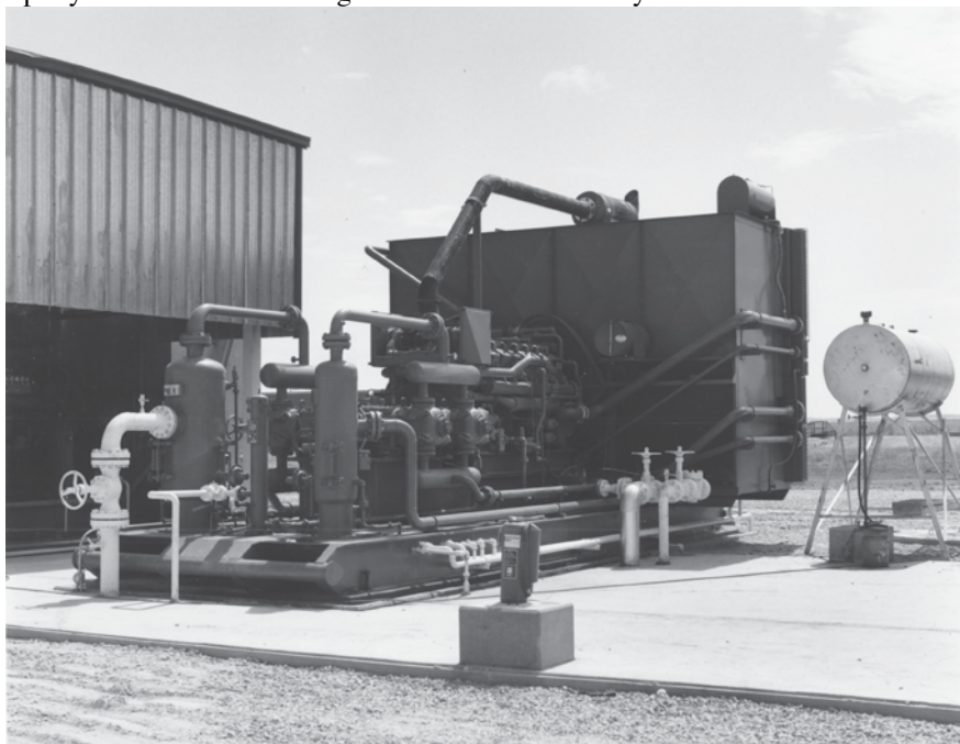
Figure 7.16 Field installation of a balanced opposed compressor in gas gathering service.
