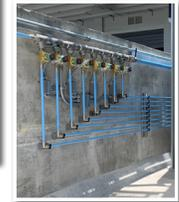
For a compressed air system to achieve maximum operating efficiency, the compressed air supply should incorporate both compressed air generation and storage. The goal is to supply the average air demand with compressors and to supply peak airflow demands from storage. The pressure of the stored air and the size of the air receiver are critical variables in managing the rate of change and properly sizing the storage.
