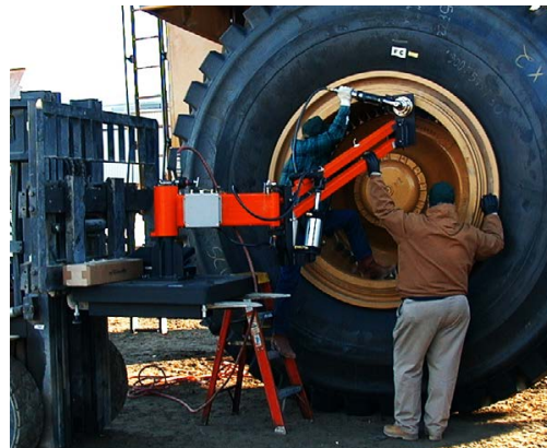
Figure 5.17: A balancer-suspended right angle nutsetter being used on construction equipment.
