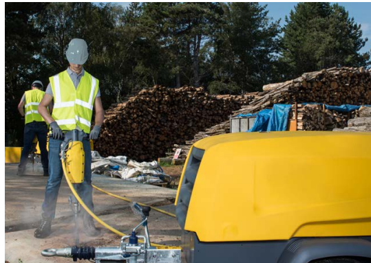
Figure 5.71: Silenced paving breaker being used on highway.
