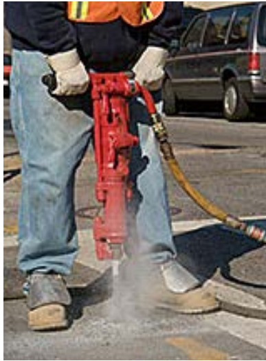
Figure 5.67: Hand-held sinker drill in the 30 to 50 lb weight range.
