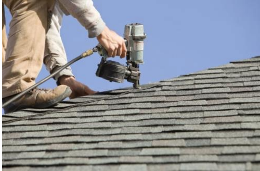
Rofer using an efficient pneumatic nail gun operating from a small gasoline powered or electric powered air compressor.
